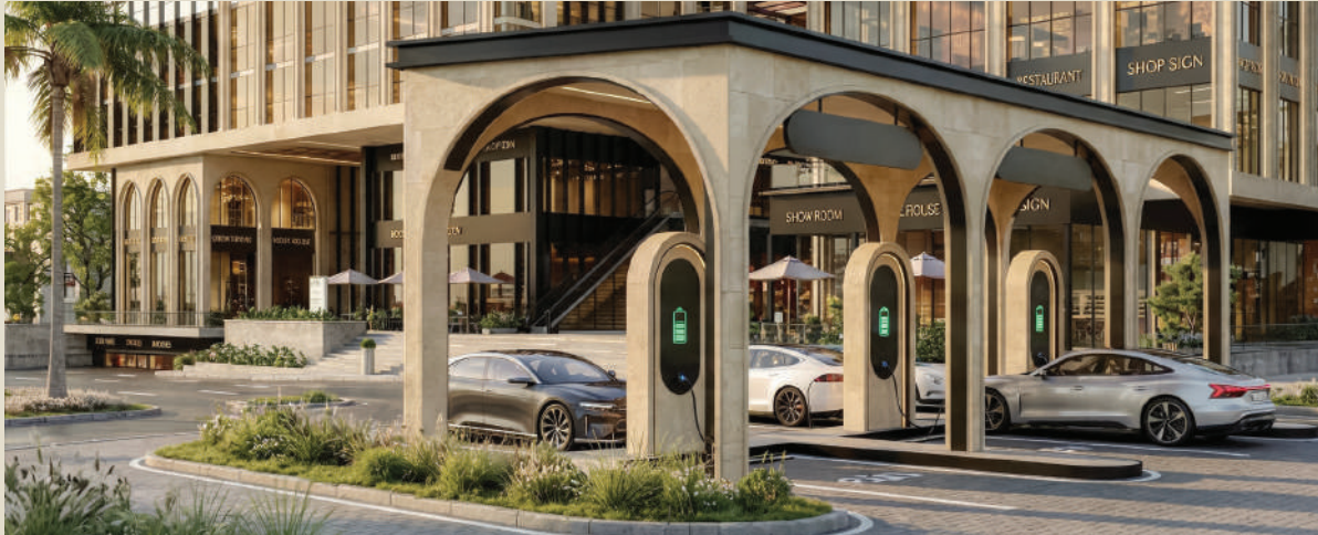
Electric vehicle charging stations
